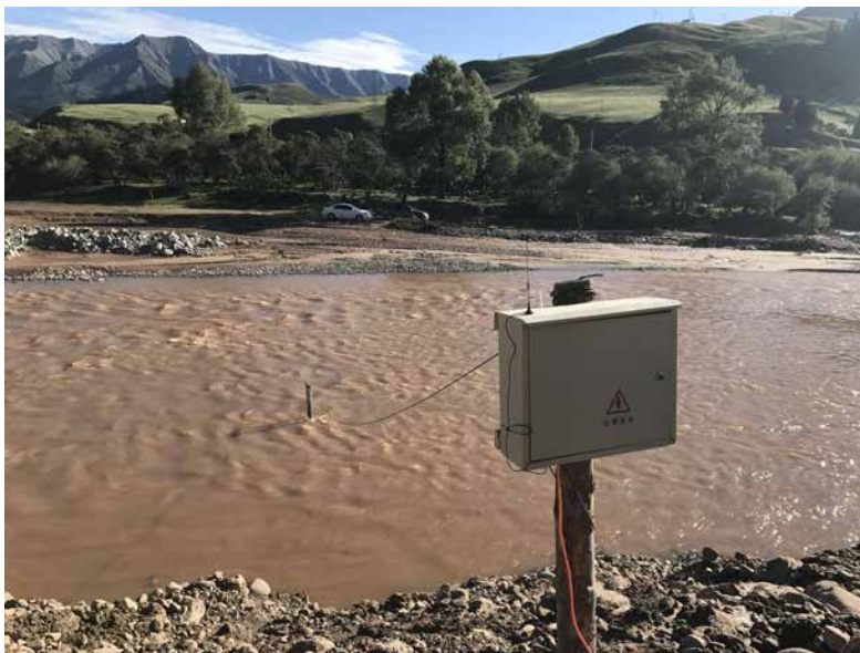
Fig. 19 Completed Installation in Wide River Channel
