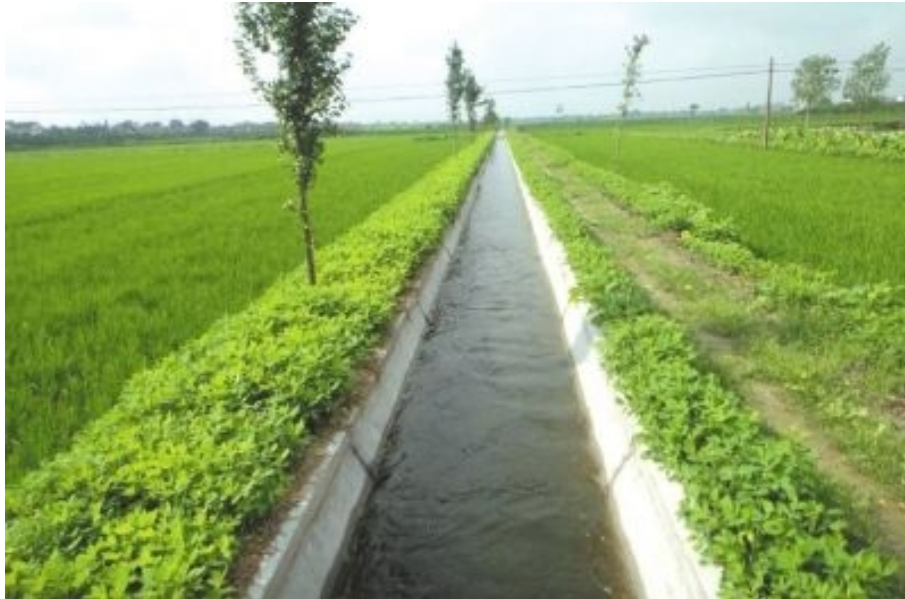
Fig. 6 Requirements for Straight Channels Upstream and Downstream of Sensor Installation
